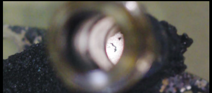
Oil supply tube. Excellent condition. Negligible deposits. No blockage.
