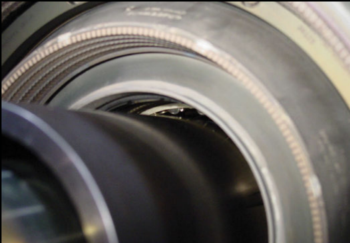
No. 5 carbon seal and bearing. Excellent condition. Negligible deposits.
